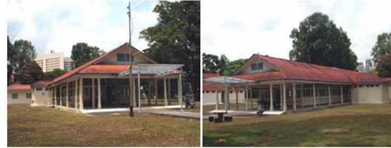
Figure H.1 Two views of the single-storey tuberculosis inpatient ward; the perimeters are free from obstruction, allowing natural ventilation throughout the year
