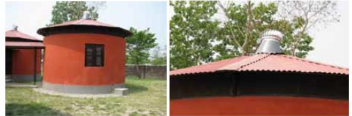
Figure 1.2 Individual isolation unit (left), and the gap between the vertical wall and the roof for natural ventilation (right)
